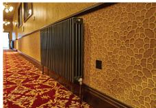
The building is heated using a gas fired condensing boiler and heat is managed in zones to make the most efficient use of energy. Each zone has been fitted with a selection of different Myson radiators which blend with the style while effectively delivering a comfortable warmth both front and rear of house.
